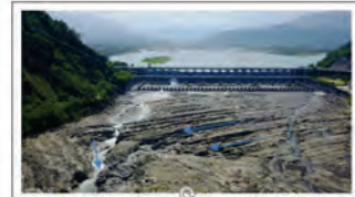
(a) Downstream of Jili Weir, ChouShui River
